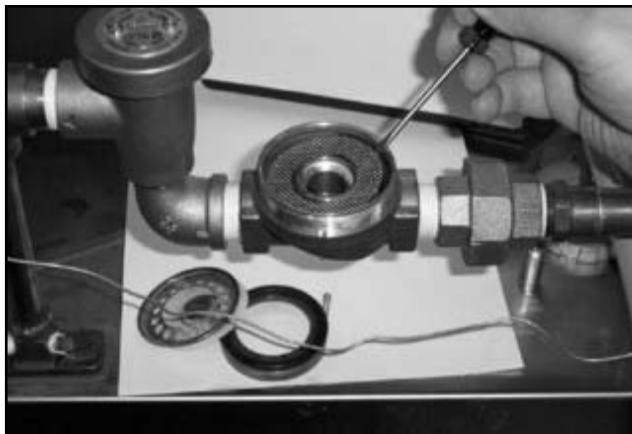
Removing the mesh strainer screen
