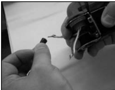
Removing the wire nuts
