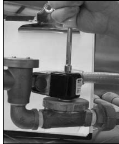
Removing the top screw
