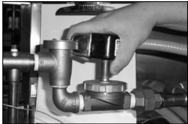
Removing the coil
