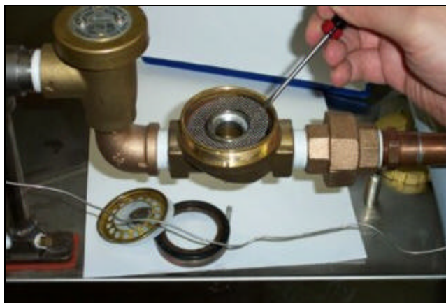
Removing the mesh strainer screen
