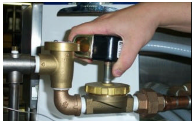
Removing the coil
