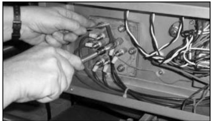
Tightening the nuts holding the power lines
