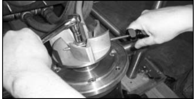
Removing the bolt that holds the impeller to the shaft
