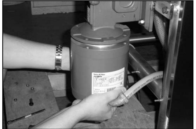
Removing the drive motor.
