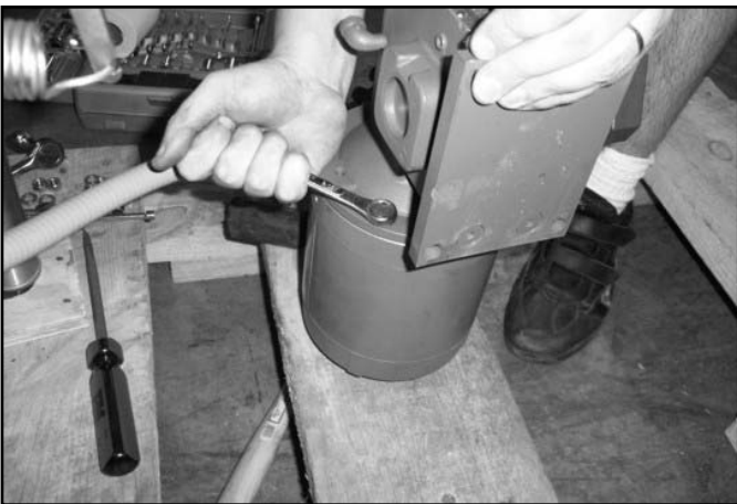
Tightening the bolts to secure the drive motor to the gear reducer.
