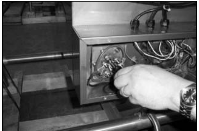
Removing the power lines.
