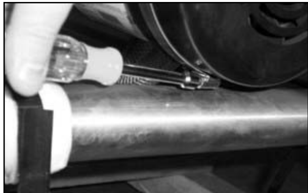
Loosening the band clamp on the back end of the motor.
