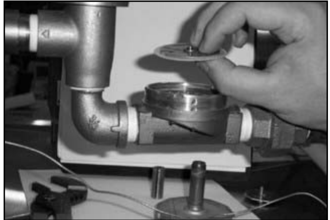
Removing the diaphragm
